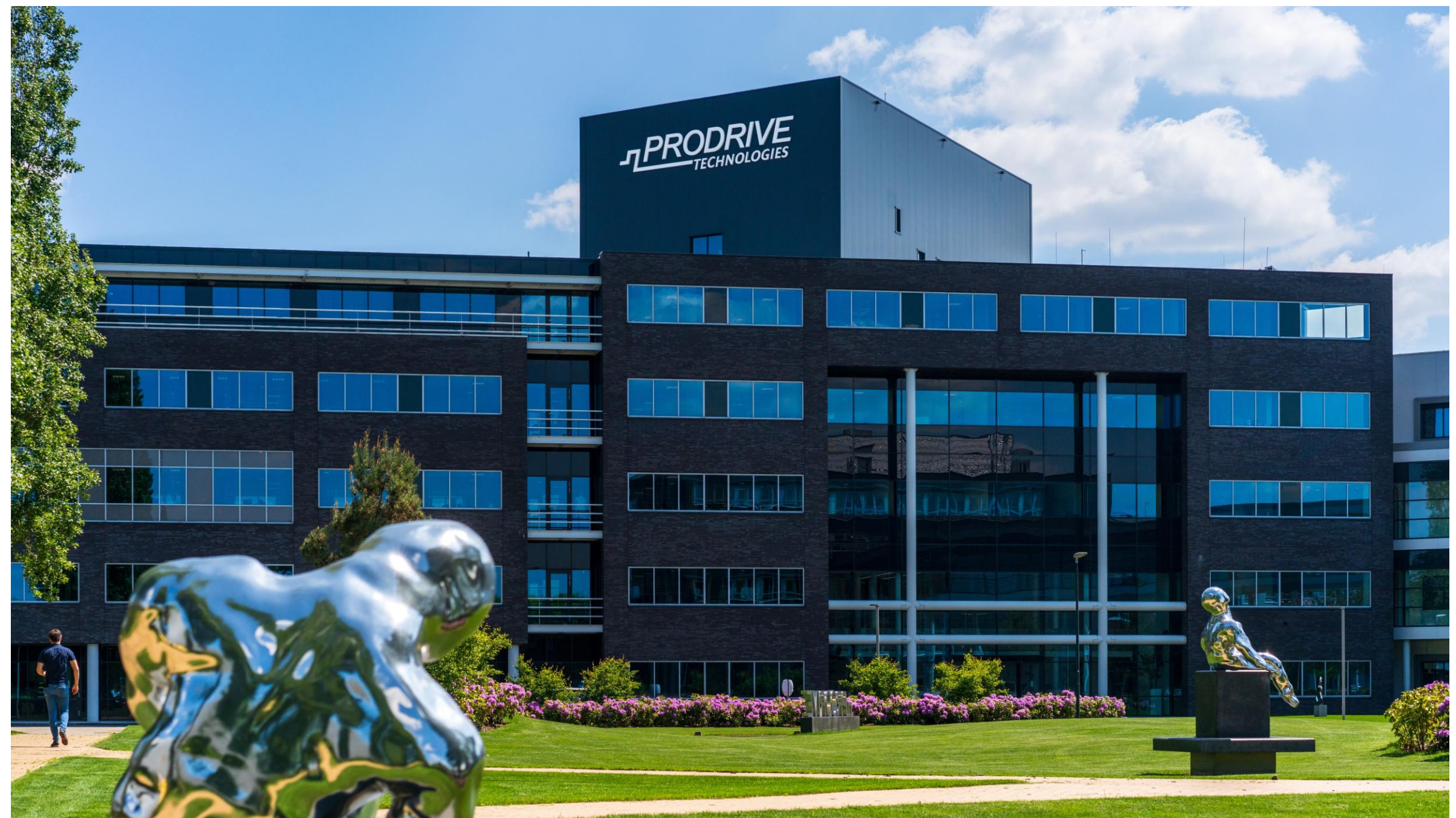
Prodrive Technologies HQ Campus, The Netherlands
