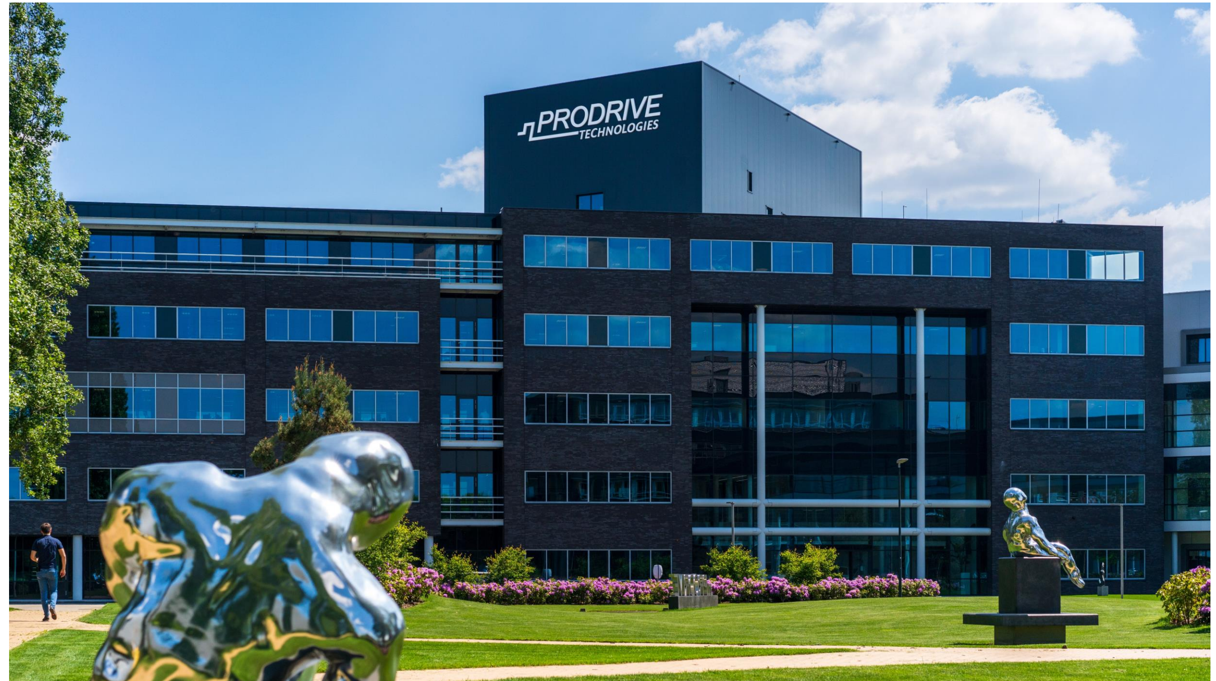
Prodrive Technologies HQ Campus, The Netherlands
